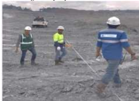
Figure 1. Blasting Area Preparation
